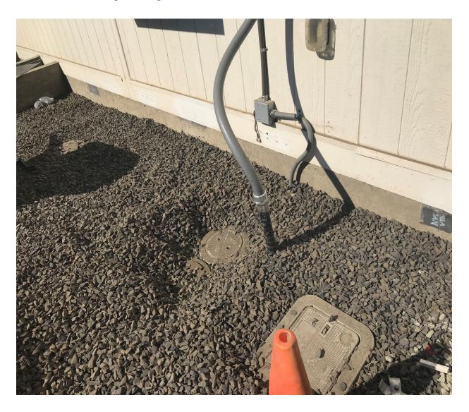
Seal all holes where previous liquid tight flex clamps were installed. Verify on all portables.
