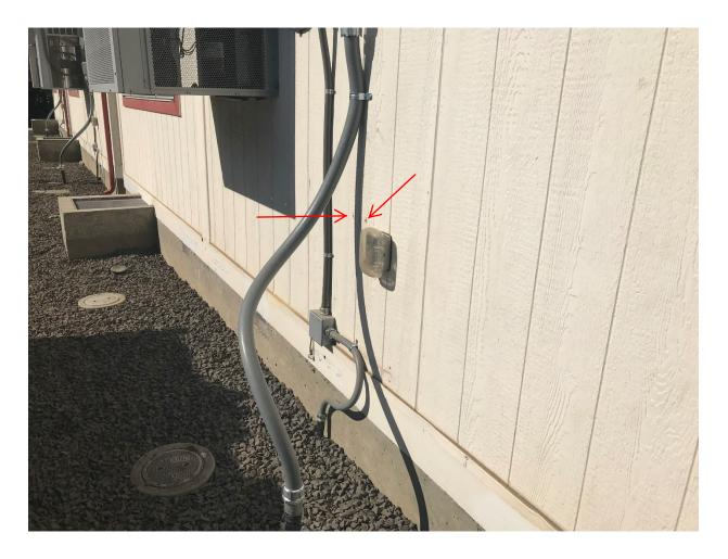
Recommend installing a new/additional clamp(s) to make installation less likely to incur any damage from externally applied forces. (No code violation).
